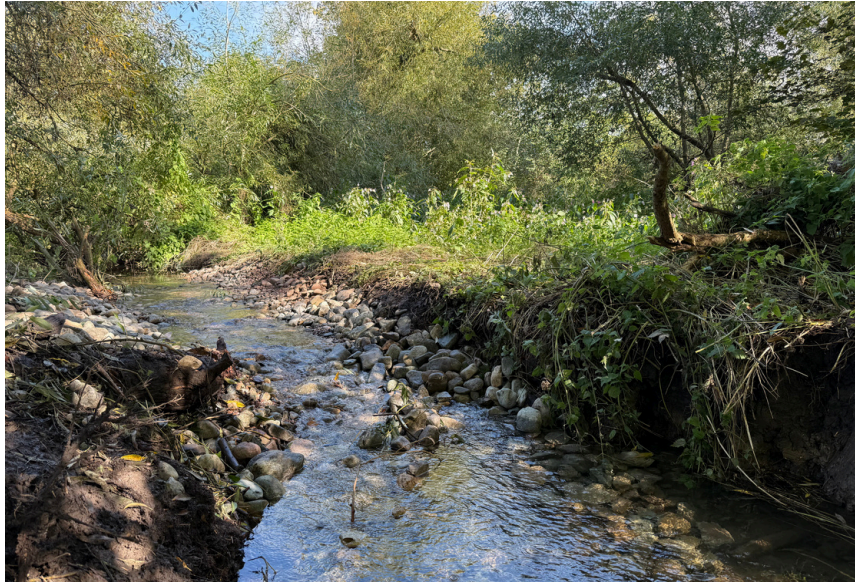
One of the sections of gravel inputted to create a riffle
