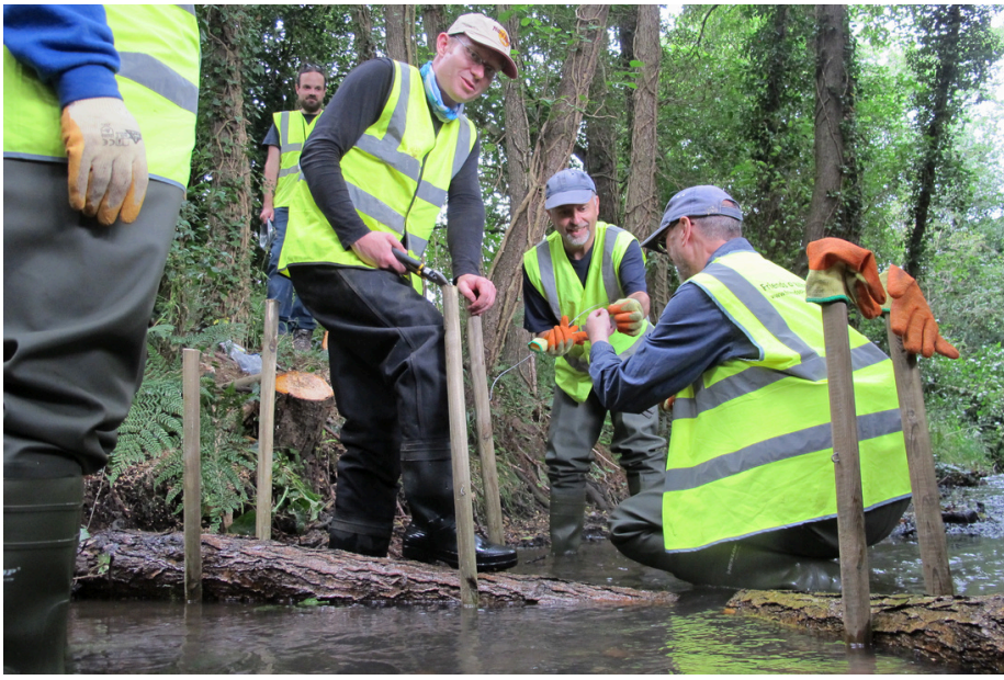
The Friends of Bilbrook within the brook securing large wood to vary flow
