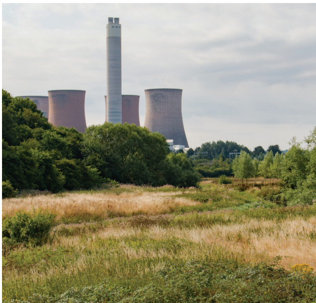
Rugby power station (Aimee L. Booth)
