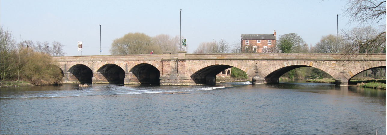
Bridge over the River Trent (Nick Mott)
