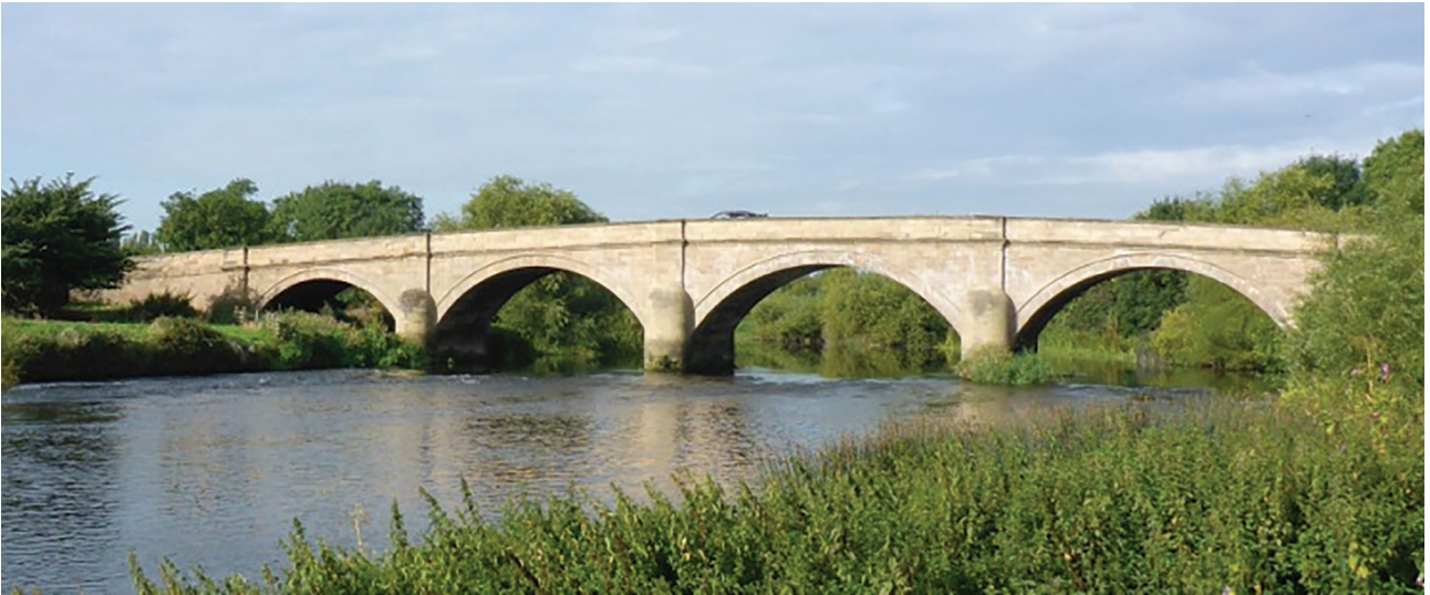
The medieval Swarkestone Bridge, Derbyshire ( ArcHeritage, 2017 )
