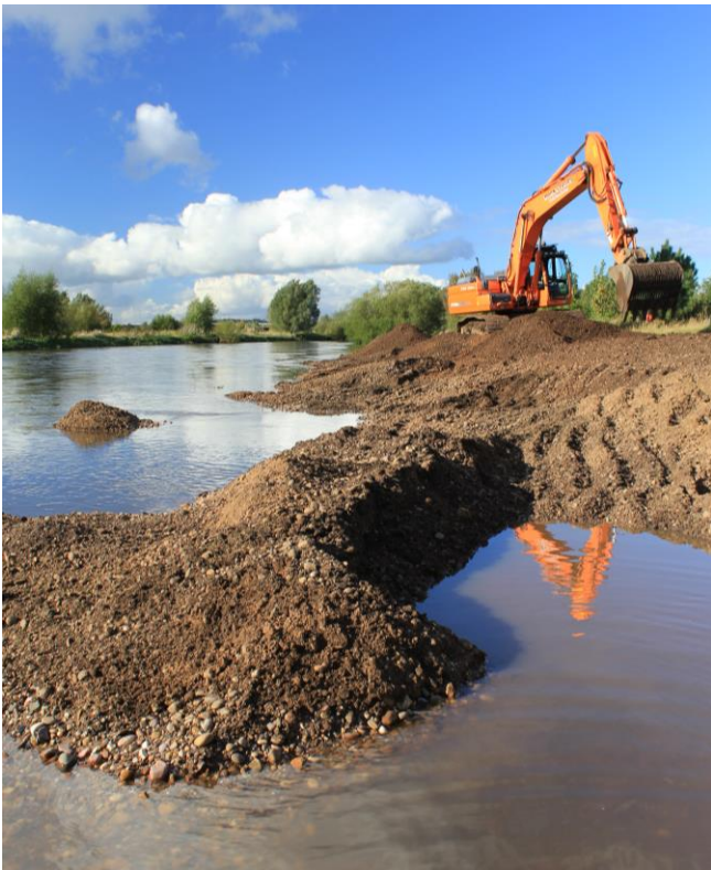
Starting work on the ground (Nick Mott)
