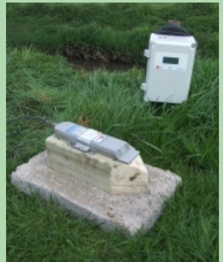
Starflow and mounting prior to installation
