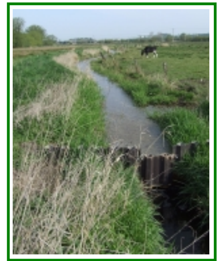
Plastic sheet piling dam raising water levels on Seighford Moor
