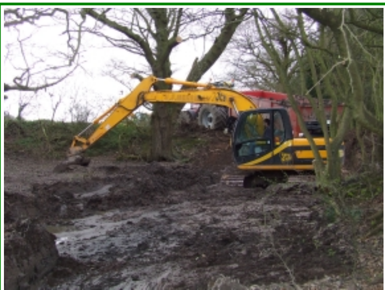
Removing silt from eastern pond
