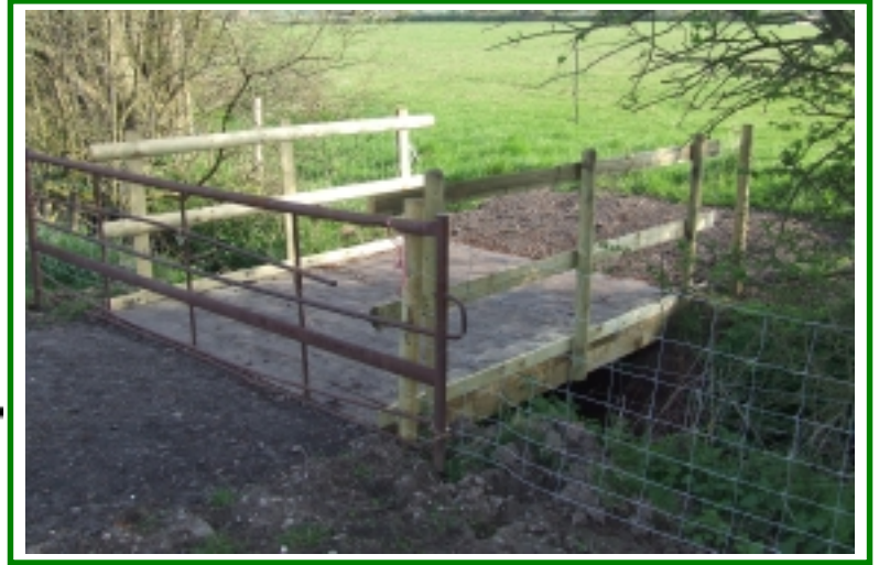
New stock bridge
