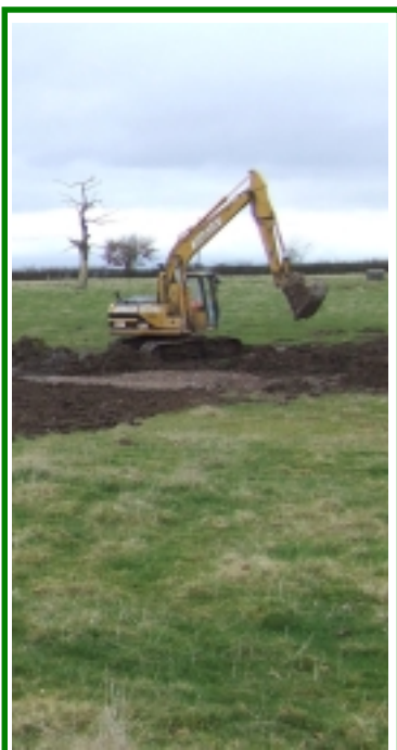
Works in progress
