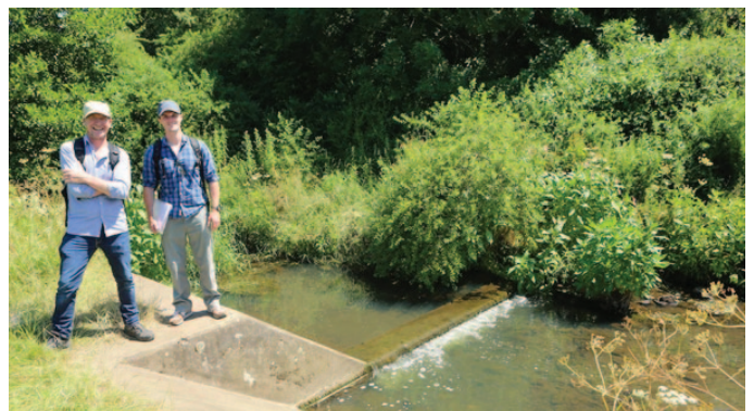
Paul and Richard visiting a weir due for removal at Cromer Road, Stoke.
