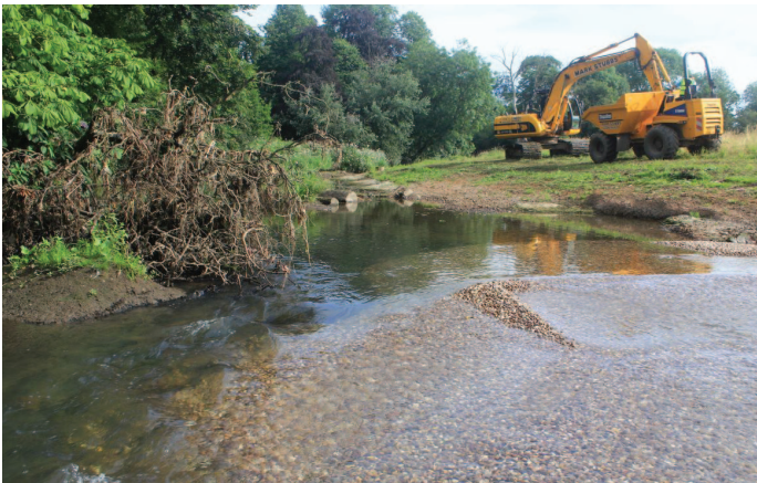
During the work
