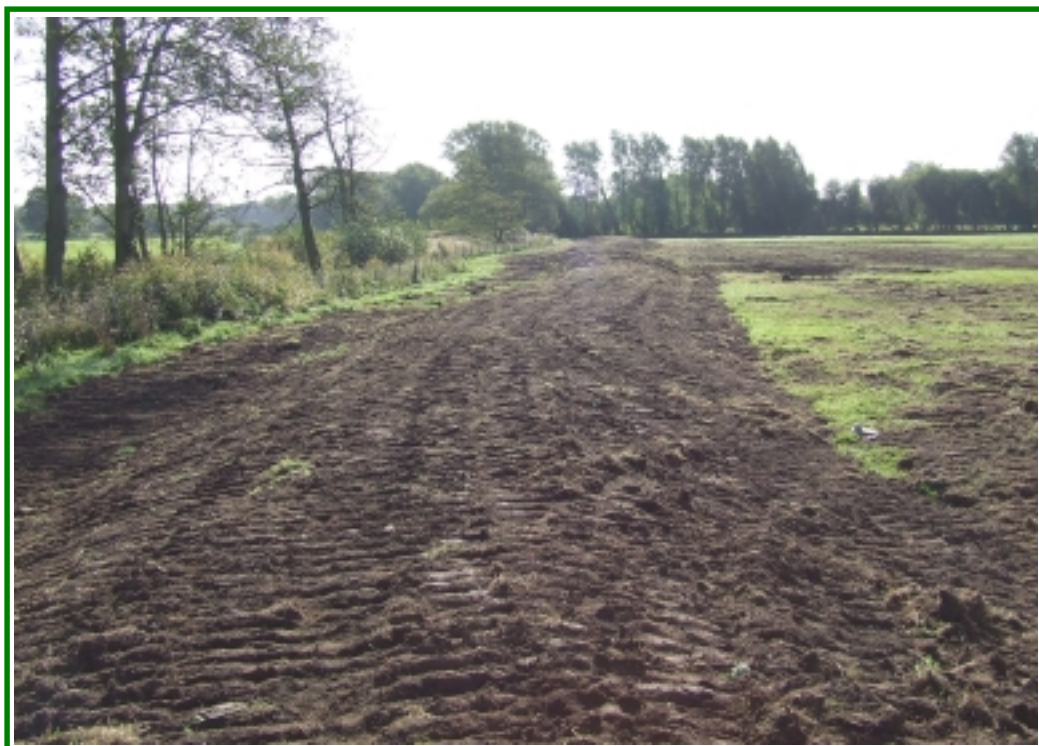
Bund adjacent to Church Eaton Brook
