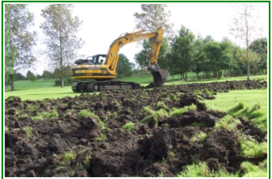
Re-profiling of fairway in progress
